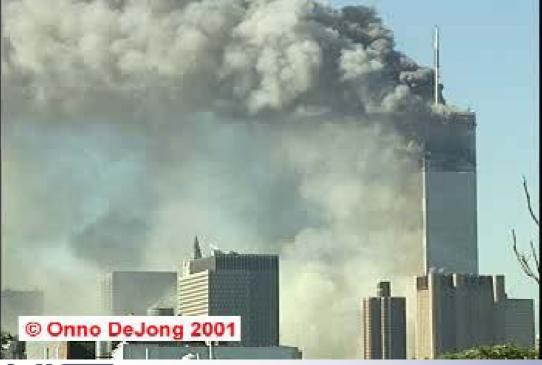
Initiation of global collapse was first observed by the tilting of building sections above the impact regions of both WTC towers.
